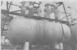
This drum is part of new smokeless tip system.
